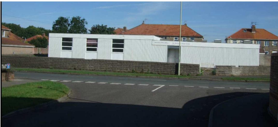
Figure 3 – Photographs of the existing application site
