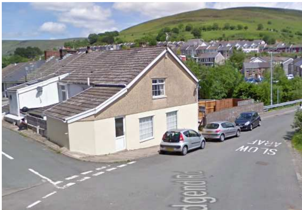
Figure 2 – Side elevation of 1 Railway Terrace
